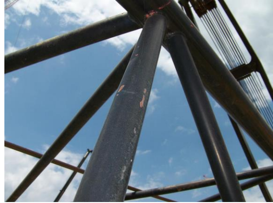
Picture of dents in the lacing in the first section.
